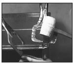
8. Use a mallet to seat the frame onto the duct.
