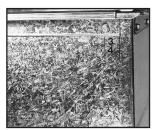
11. It is essential that the frame angle is fastened to the duct within ¾" of the end of the angle at each corner.
