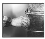
Carefully align mating frames before they touch. Ductmate 440 adheres on contact. A drift pin can be used to correct any misalignment.
