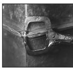
18. Compress gasket at corners with vice-grip while snapping in corner clips.
