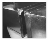
16. On the mating Ductmate frame apply 440 gasket only to the corners as in photo (approximately 3" per corner). The same 3 point application requirements apply as in photo 14.
