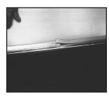
Apply 440 gasket completely around Ductmate frame to the beginning point. Where gasket meets overlay about 3/8".
