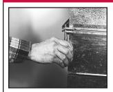
Align duct sections to be connected. Bolt duct sections together at all four corners using 1" x 3%" bolts for the Ductmate 35 system and 1" x 5/16" bolts for the Ductmate 25 Systems. Do not use the Ductmate "no bolt clips" for removable duct applications.
