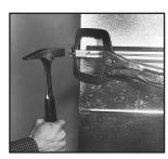
Slide corner clips onto the Ductmate 25/35 joined corner pieces. Tap with hammer until rear tab clicks into notch on corner pieces and locks in for a permanent connection.
