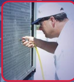
Blow off coils with Sludge Sucker® Blowgun
