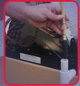
Clean out condensate drain lines with Sludge Blaster®
