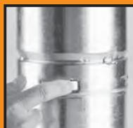
Depress the SureLock™ tab to secure pipe sections.
