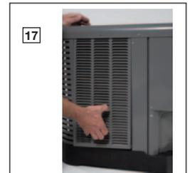
The outdoor fan motor has sleeve bearings and is inherently protected. The motor is totally enclosed for maximum protection from weather, dust and corrosion. (18) Access to the outdoor fan is made by removing four fasteners from the fan grille. The outdoor fan can be removed from the fan grille by removing 4 fasteners in the rare case outdoor fan motor fails.
