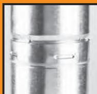
Push the ends of the pipe together.
