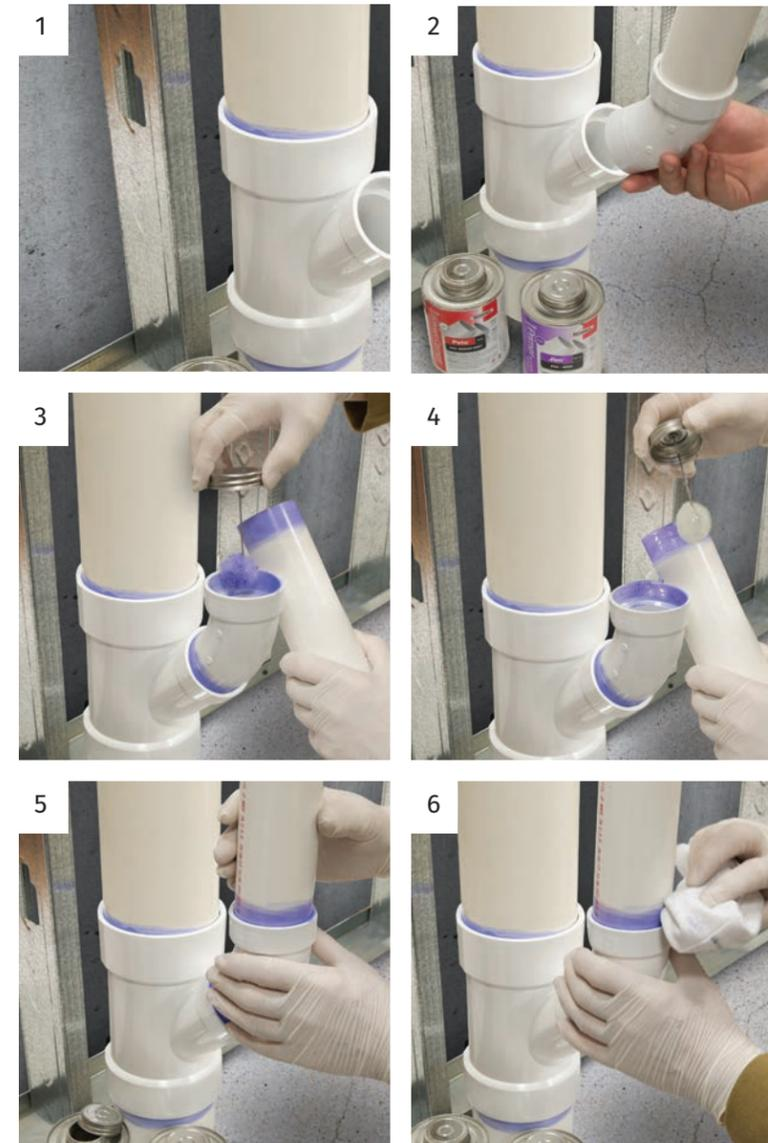
1. Needed to make weld - Pipe fittings, primer, solvent and deburring tool.
